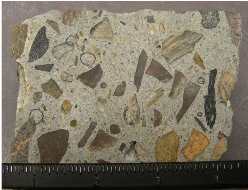
Figure 6. Lapped cross-section of a portion of core sample, top surface of concrete is on left side of photograph. A few areas were circled with a black felt-tip pen to indicate some of the numerous localized concentrations of secondary deposits.
