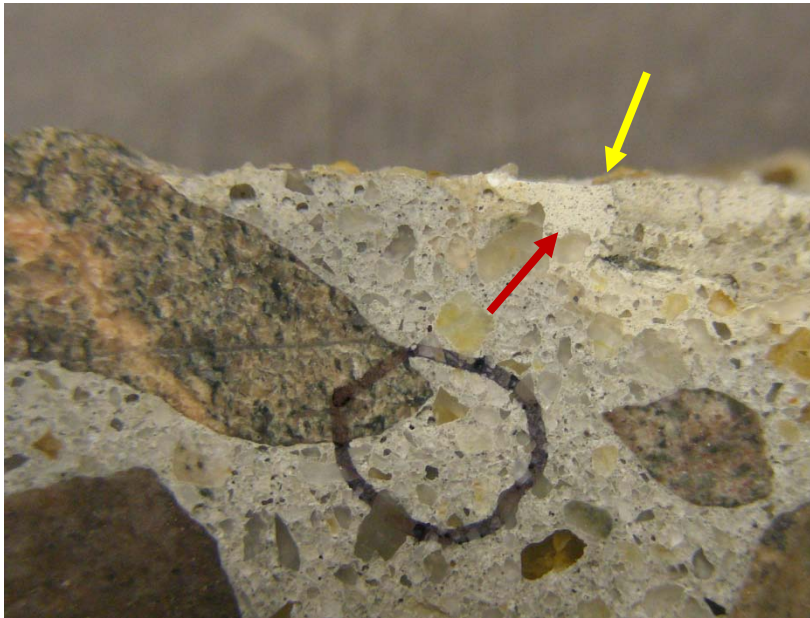
Figure 8. Near-surface zone showing a zone of deteriorated paste (red arrow). The yellow arrow indicates where paste ends and aggregate socket begins.
