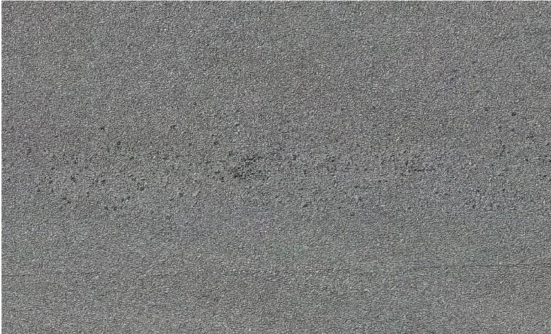
Photograph 31: Raveling (medium-severity)
