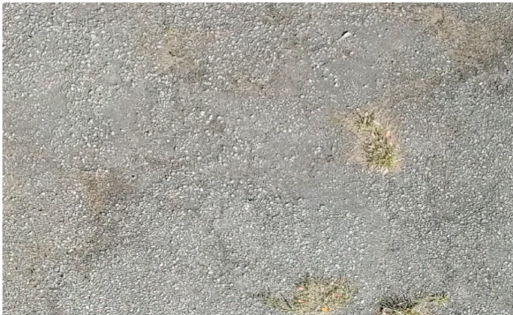
Photograph 18: Raveling (High-Severity)
