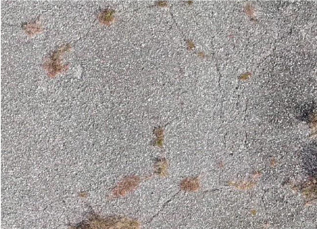
Photograph 25: Raveling (high-severity)
